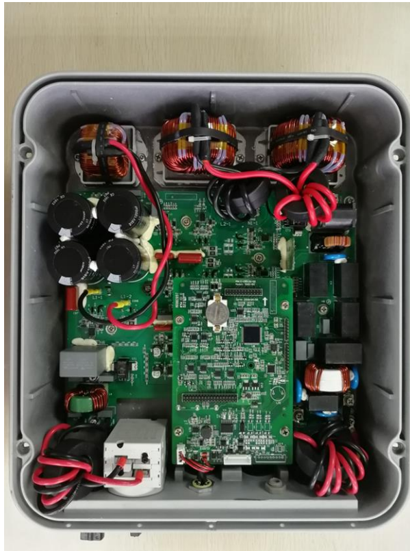
Figura 4. vista interna-1 Figure 4. Internal view-1
