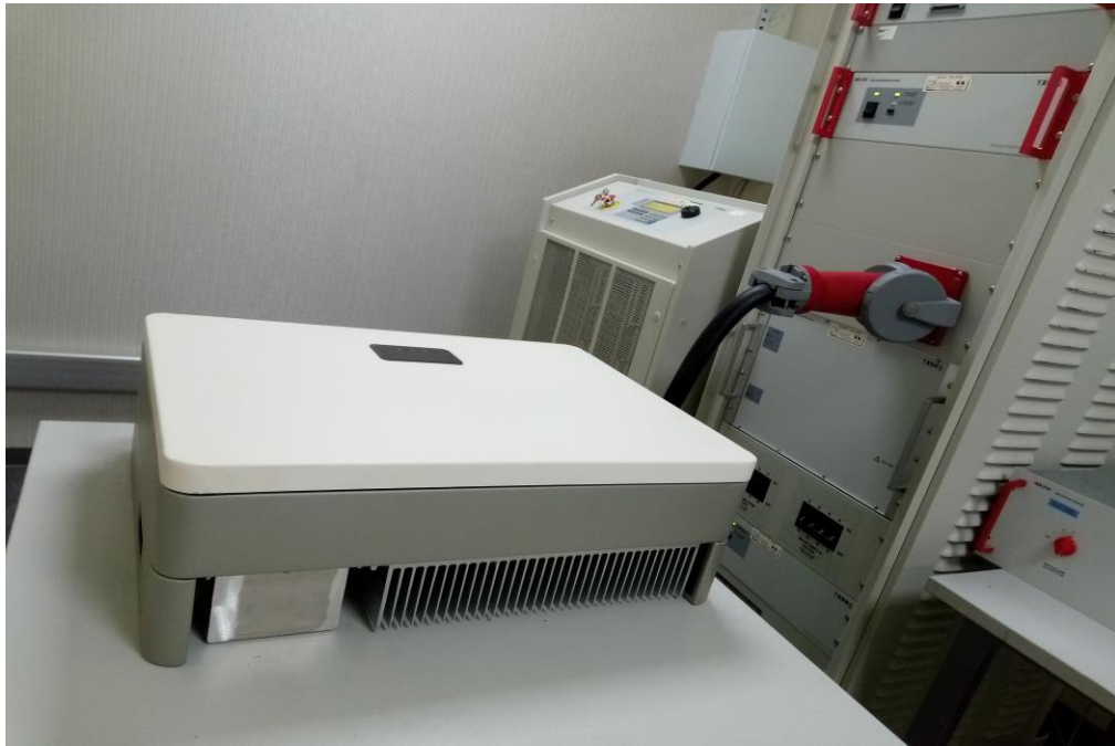
Figure 6 Harmonic current emission test setup
