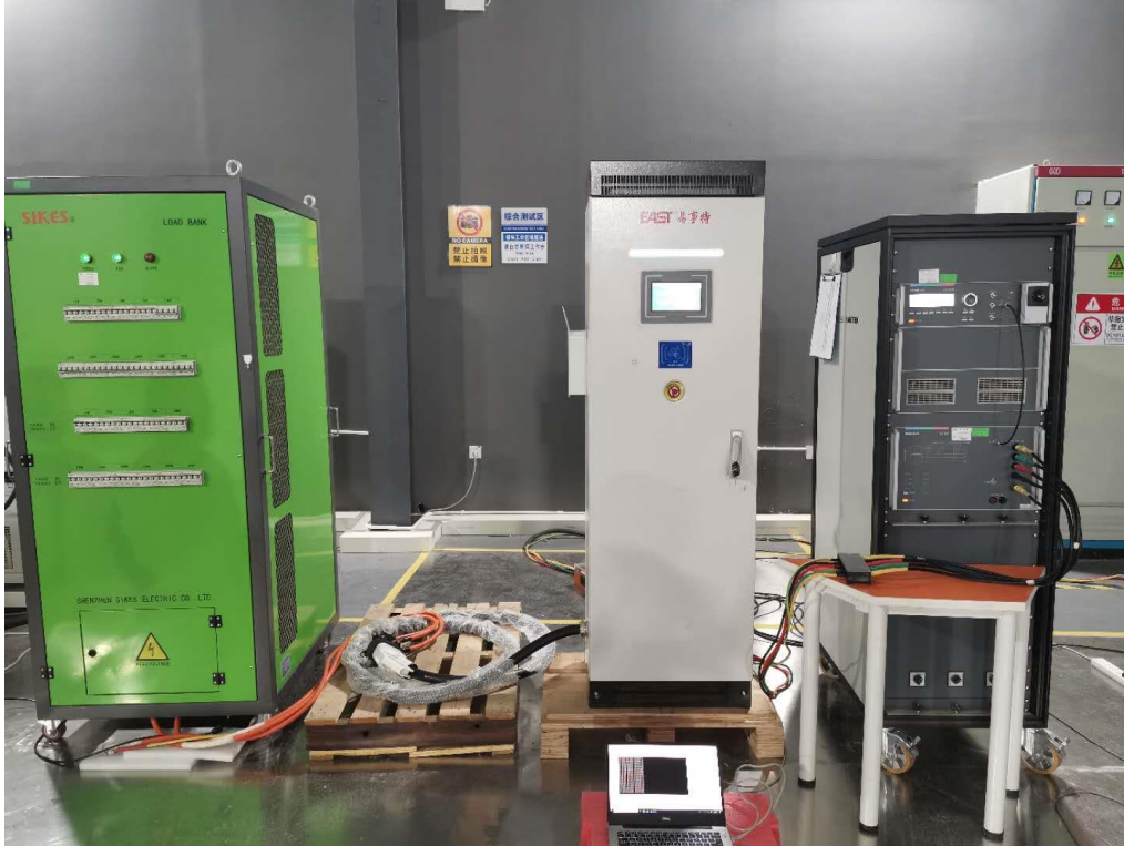
Photograph 8: Set-up for Surge (AC Power Input Port)
