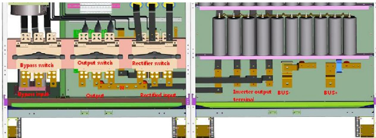
Fig. 3-37: Connection terminal of this series (400-500kVA) UPS
